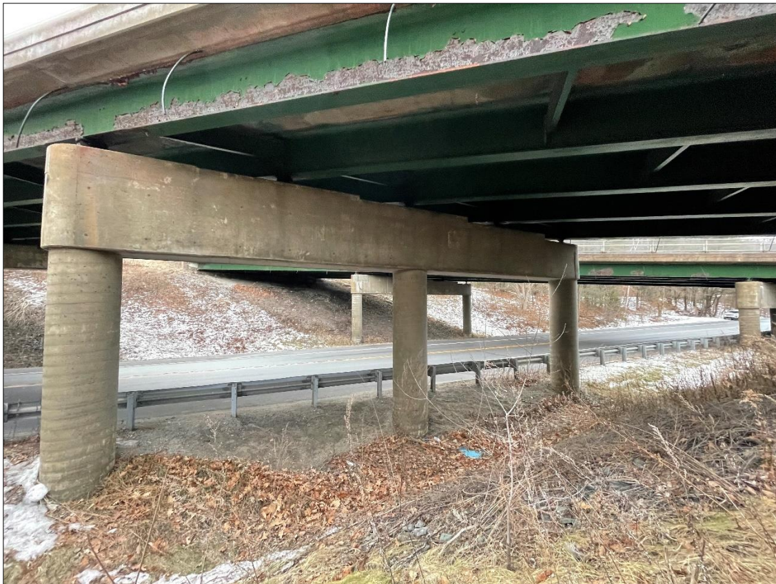
Bridge 25N Southern Pier
