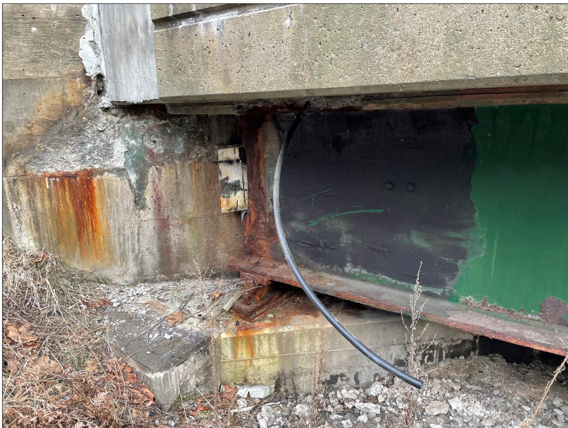
Bridge 25S Northern Abutment Western Fascia
