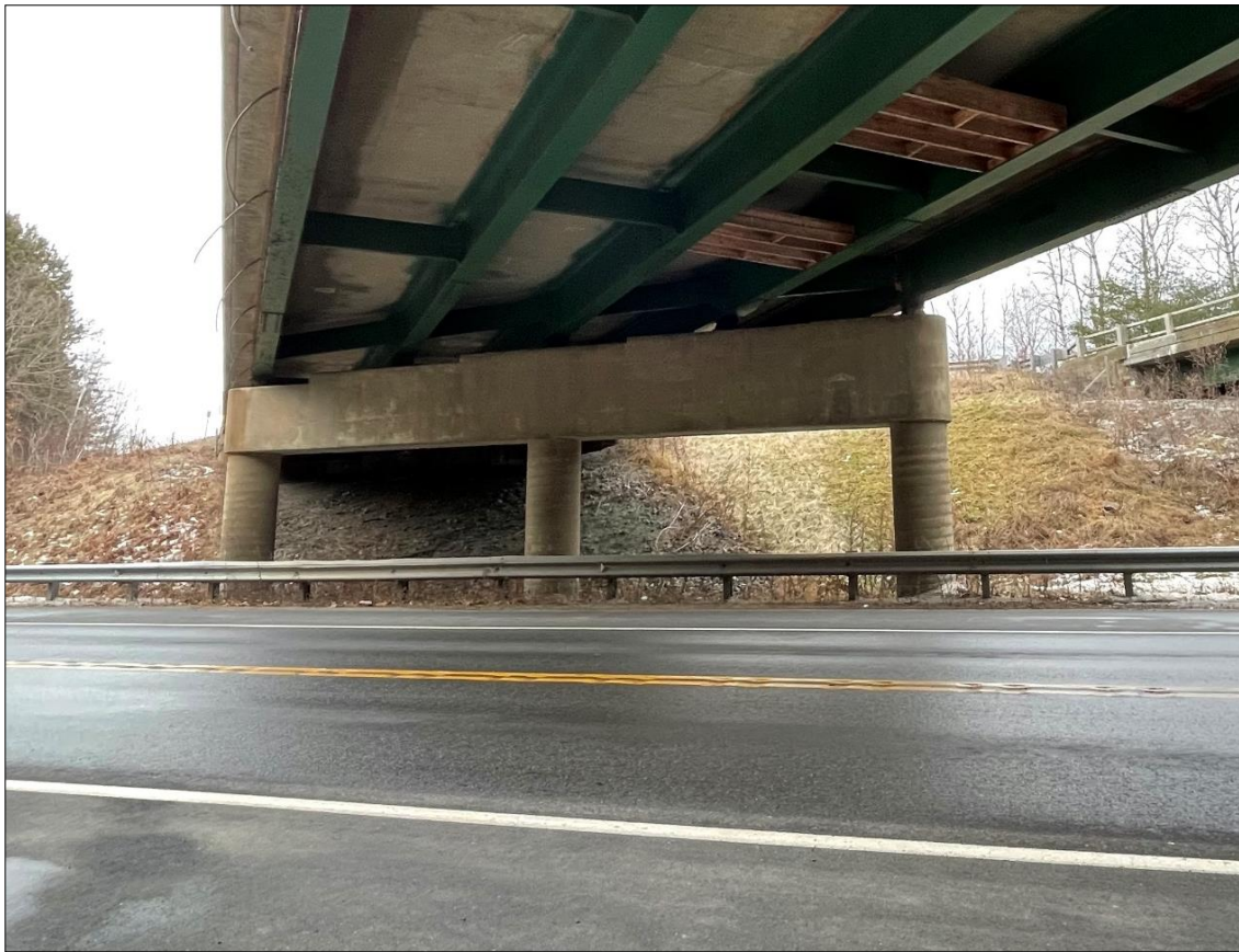
Bridge 25S Southern Pier
