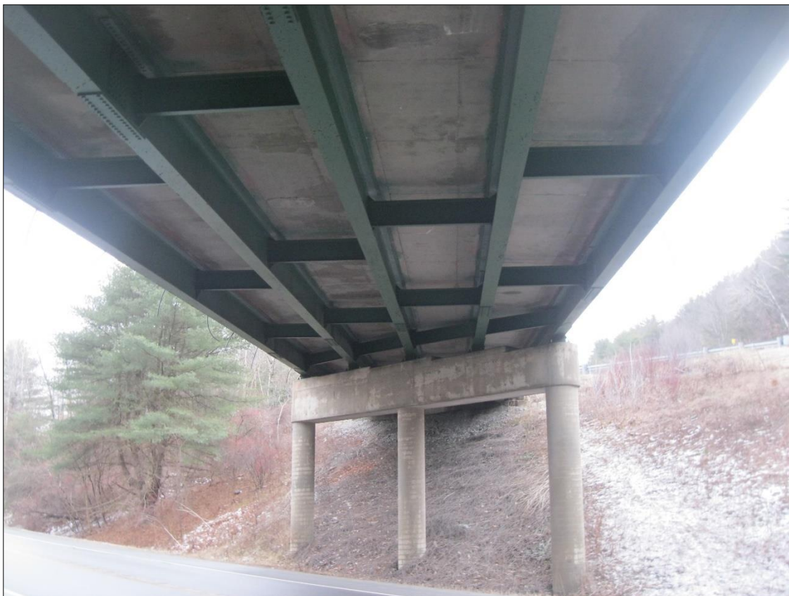
Bridge 25N Deck Underside at Midspan
