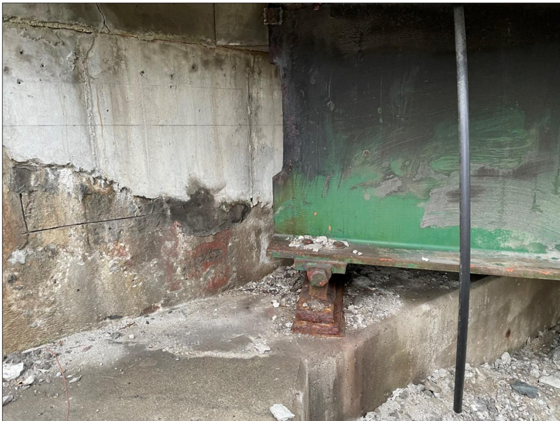
Bridge 25N, Northern Abutment Eastern Fascia
