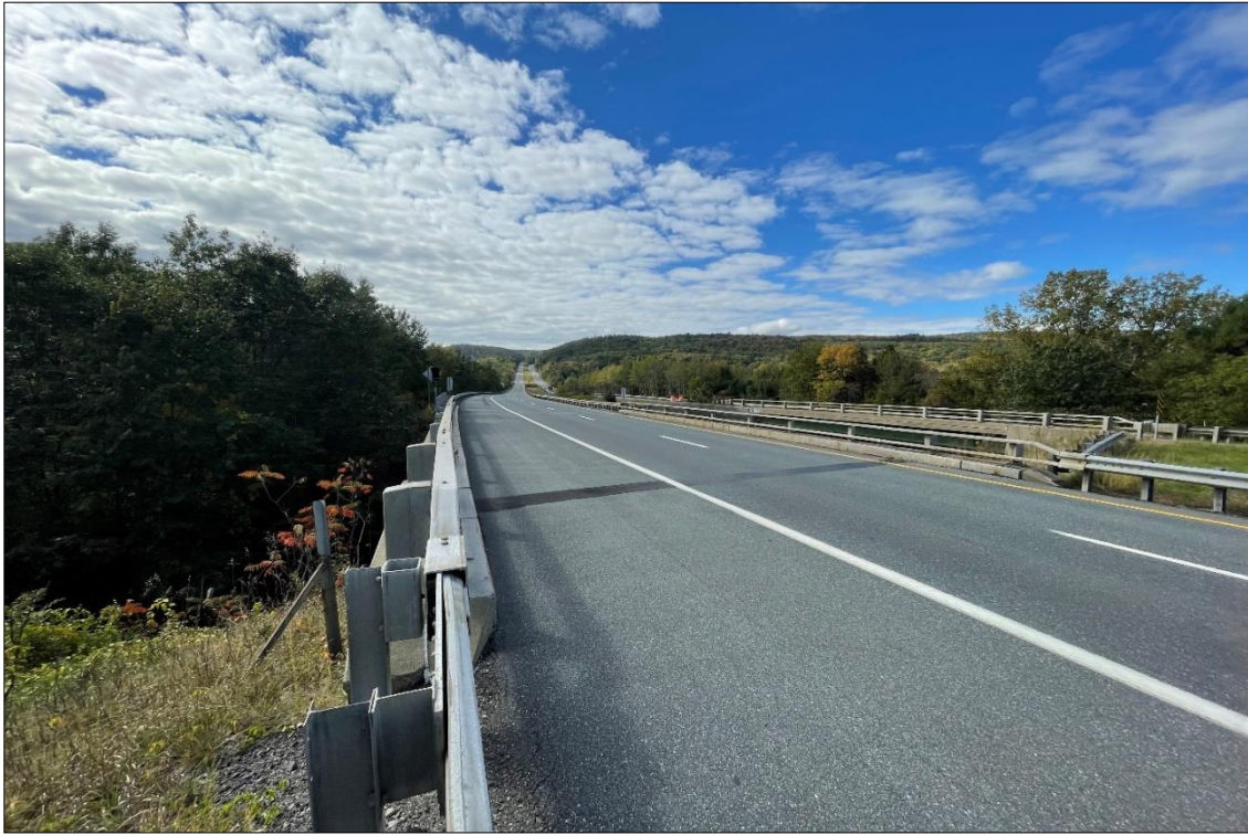
Looking north over Bridge 27N
