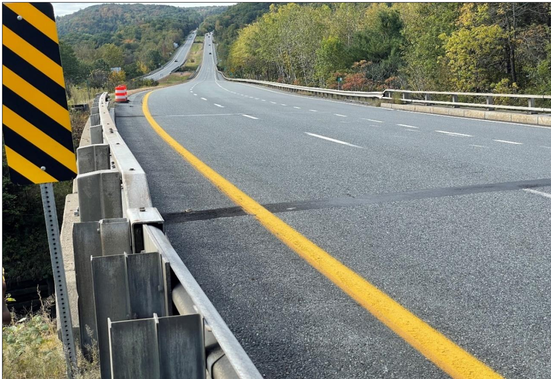
Looking South over Bridge 27S
