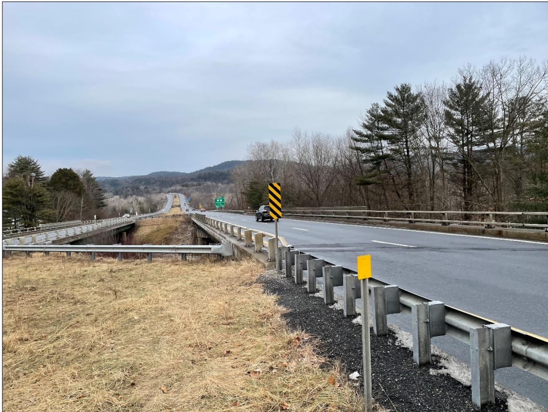
Looking South over Bridge 25N
