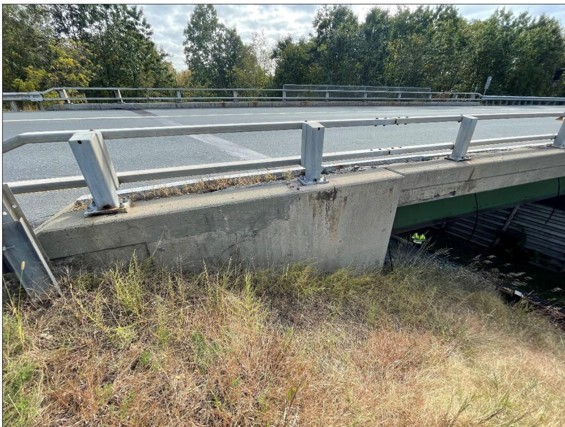
Bridge 27N Wingwall and Deck End
