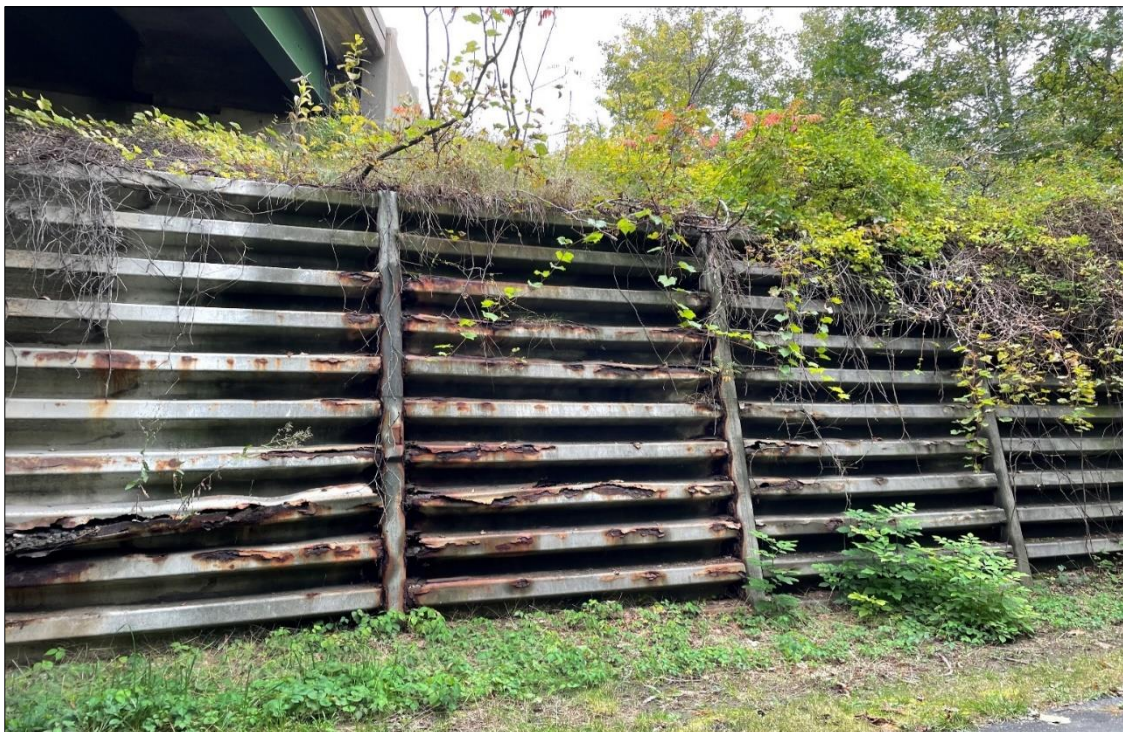
Northern Bin Wall Under 26S Median Fascia
