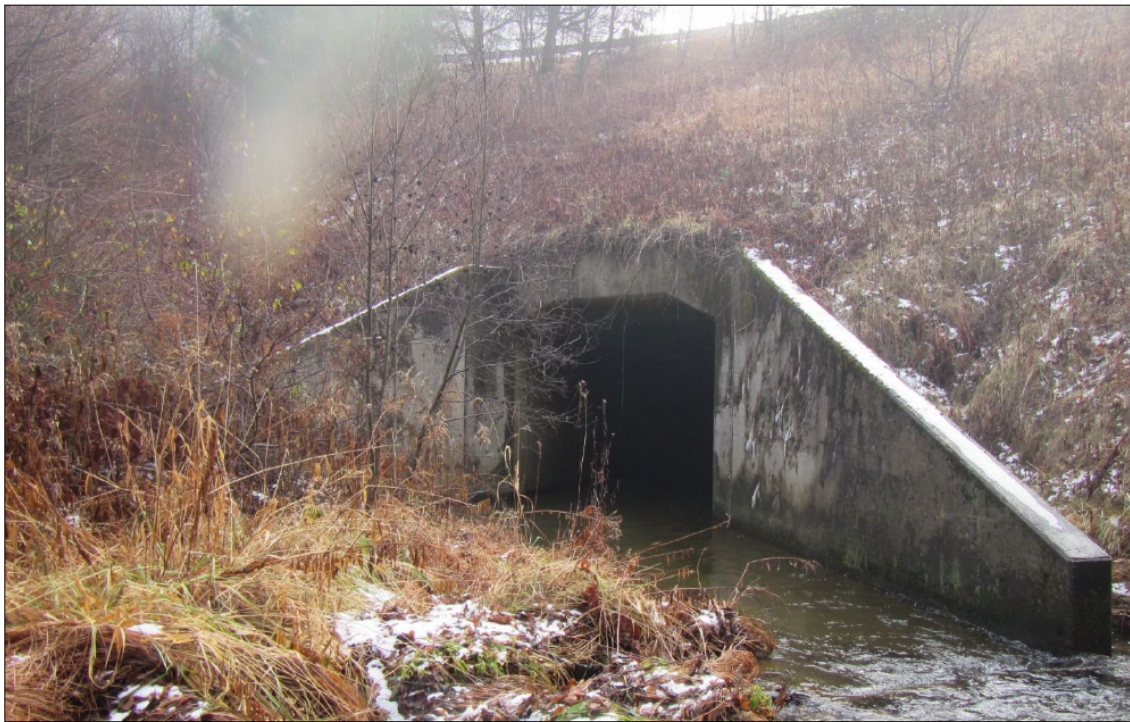
Spencer Brook Culvert and Exit 7 Ramp
