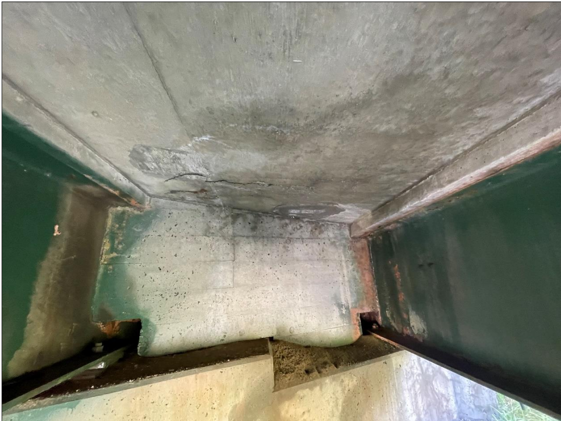
Bridge 27N Abutment Backwall and Seat
