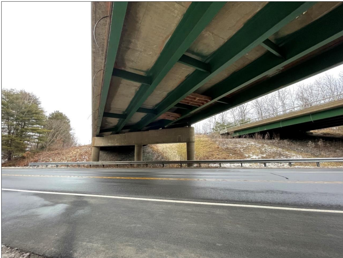
Bridge 25S Deck Underside at Midspan
