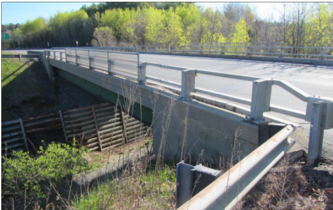
Bridge 27N Median Fascia
