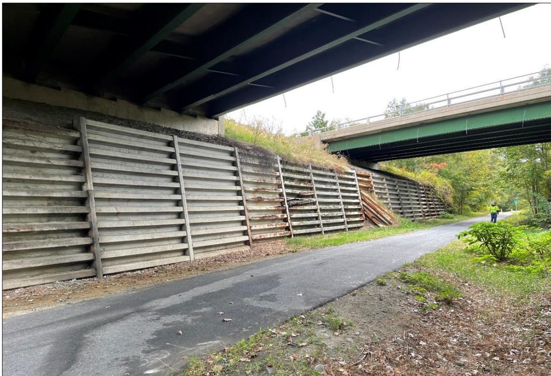
Northern Bin Wall
