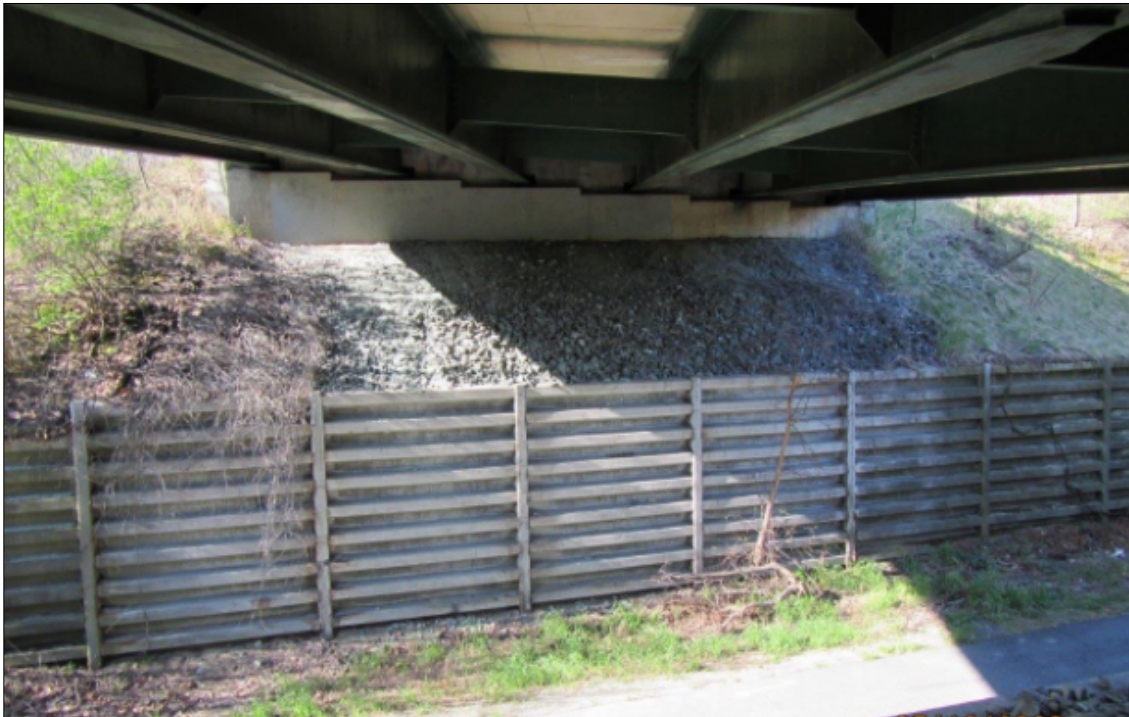
Bridge 27N Abutment and Bin Wall
