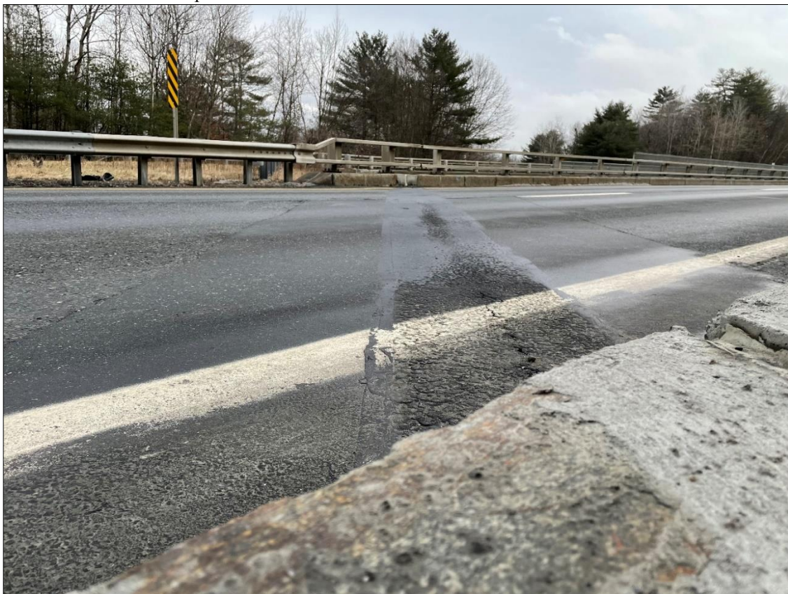
Bridge 25S Northern Deck Joint
