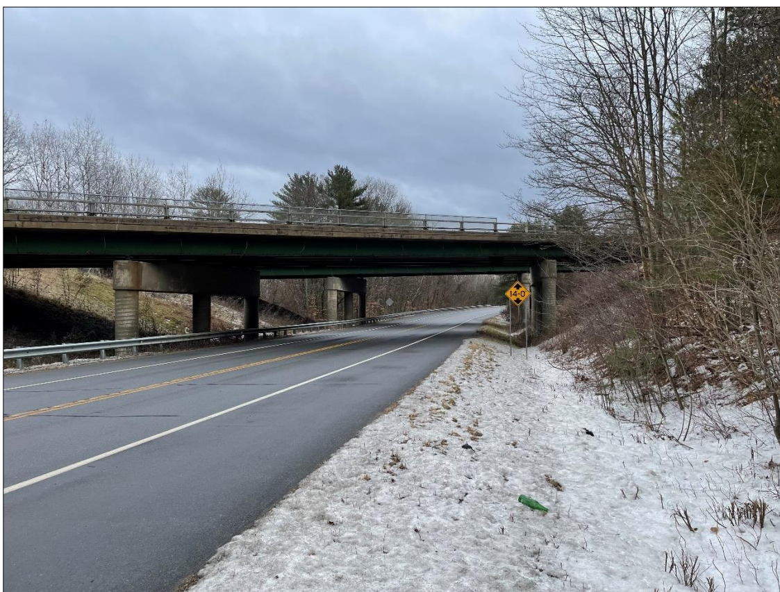
Bridge 25S from Route 5 Looking East
