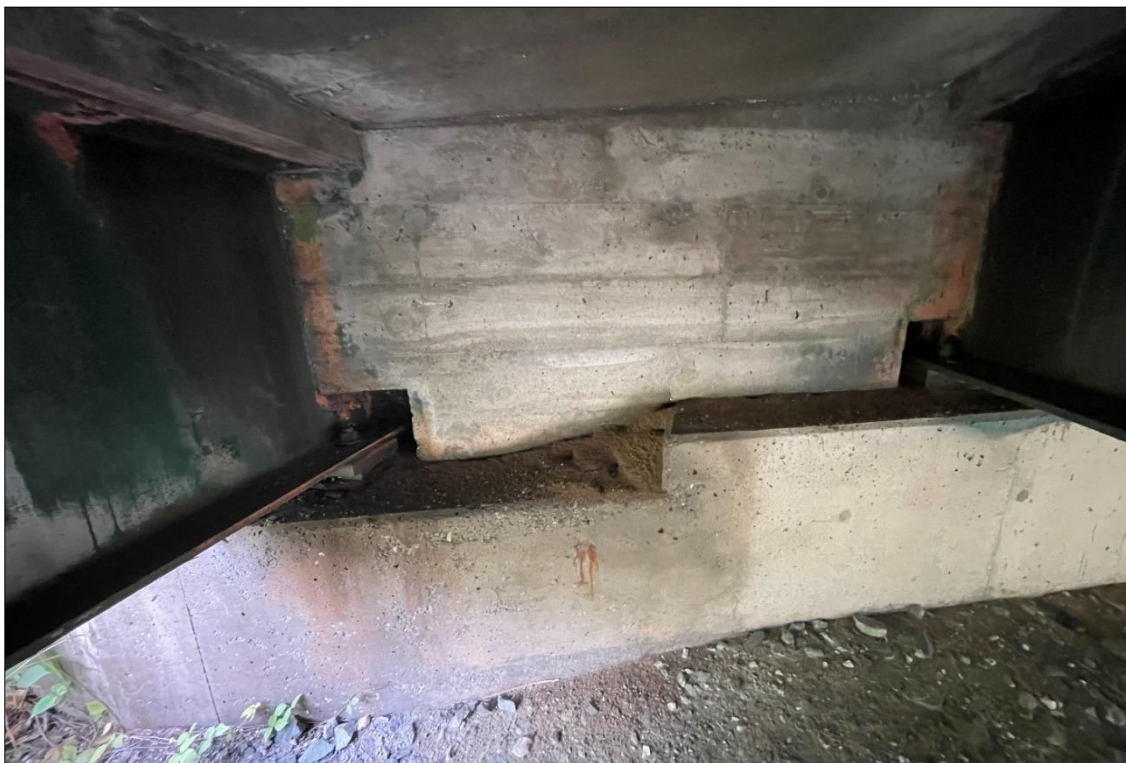
Bridge 27S Abutment Backwall and Seat
