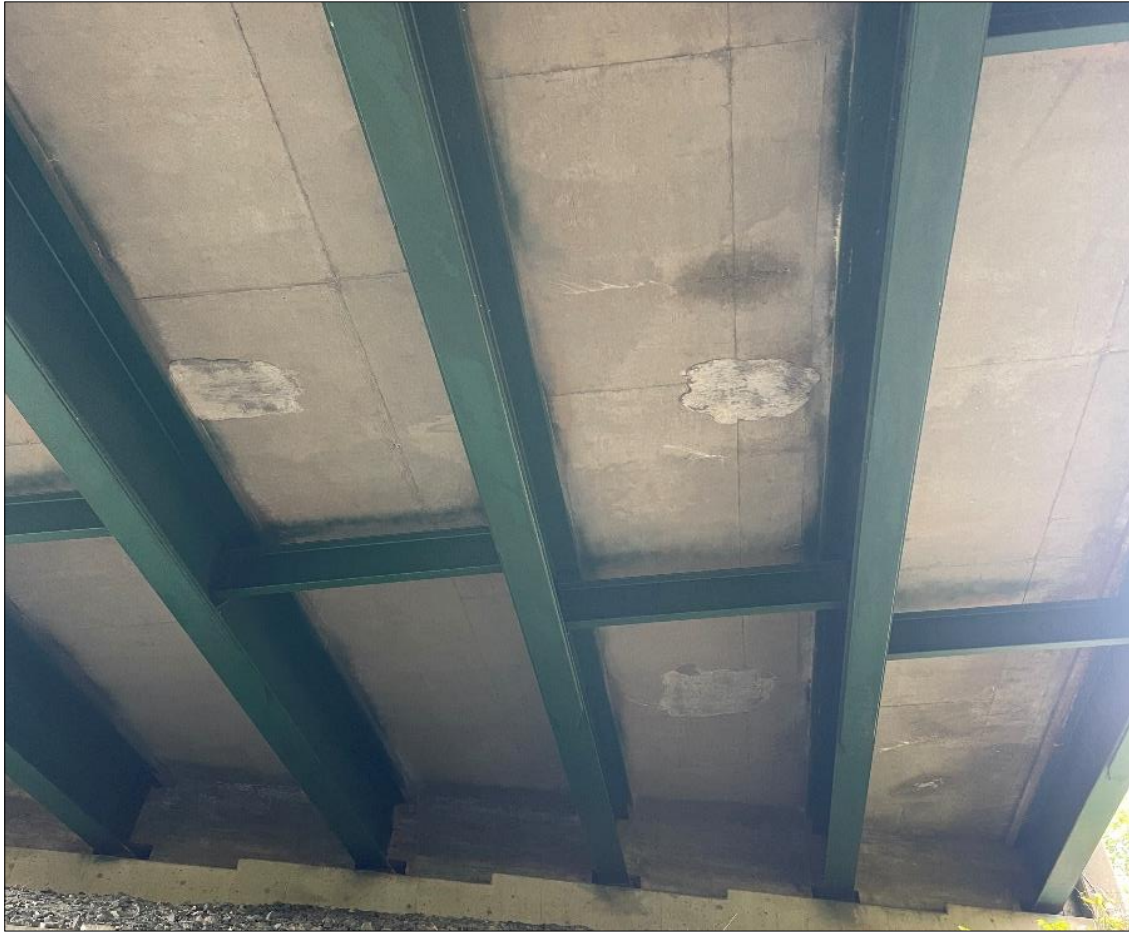
Bridge 27N Deck Underside at Abutment
