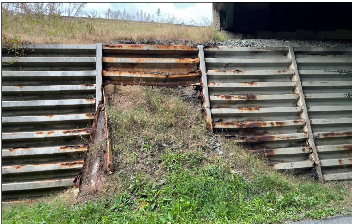
Northern Bin Wall Under 26N Median Fascia
