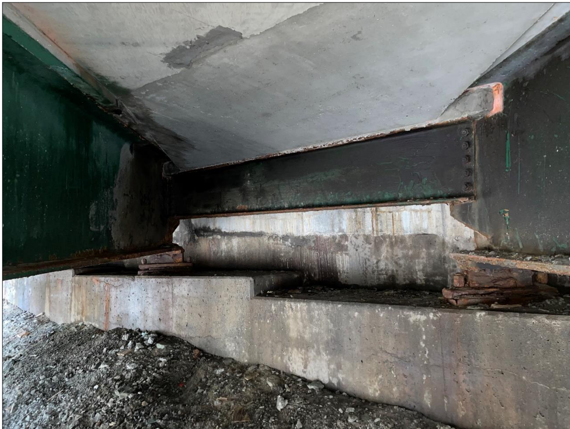
Bridge 25S Southern Abutment and Bridge Seat
