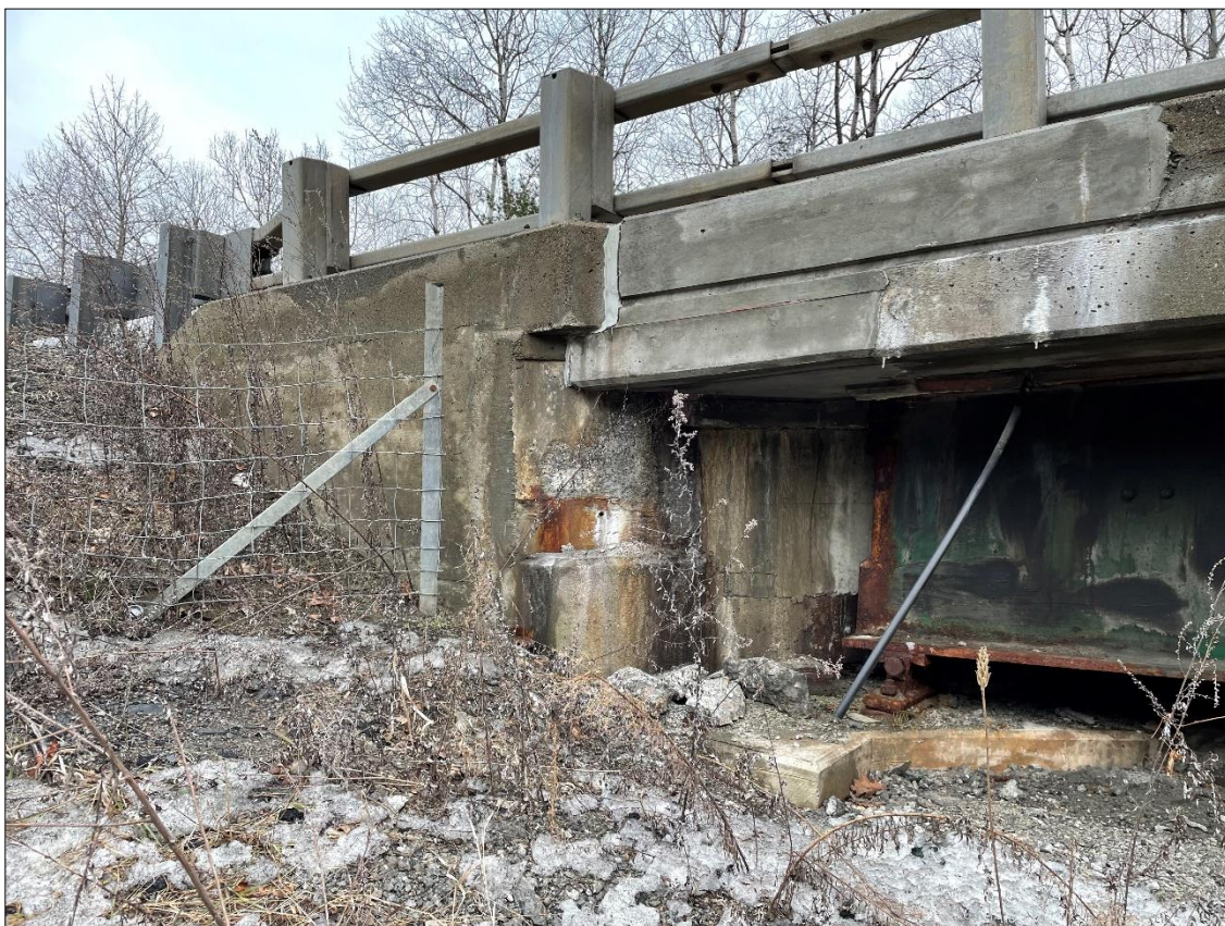
Bridge 25N Northern Abutment Western Fascia
